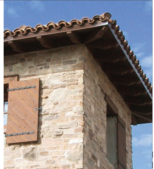
LEFT: The tile blend labeled 'Custom' is the fourth and perhaps most attractive blend of the Boral/Monier LifeTiles Barcelona S-Tile project. Hand-blending 3 other colors in the field created it.
